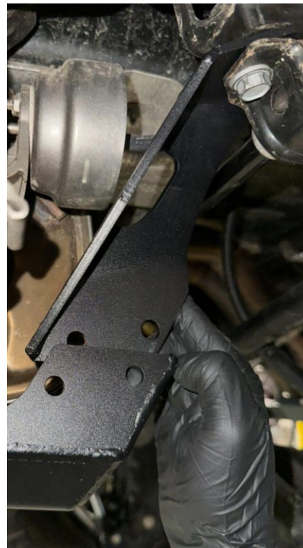
Figure 8: Passenger side rear support bracket loosely installed
