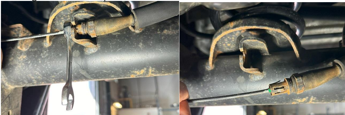
Figure 2: Emergency brake cable housing in axle bracket and then removed
