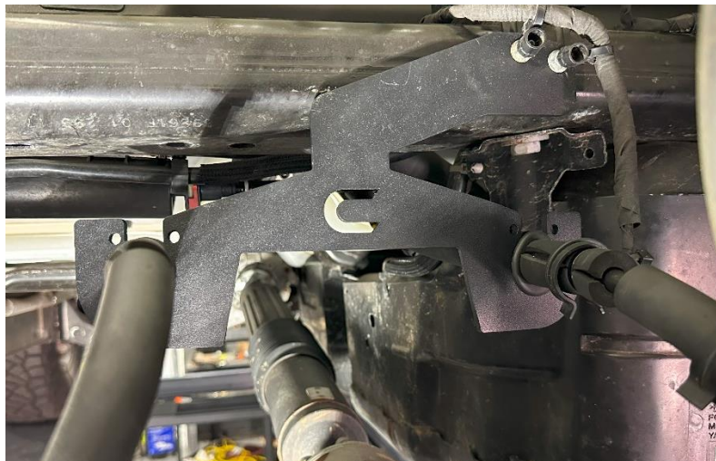
Figure 7: Cable housings installed
