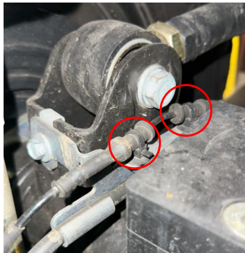
Old ABS zip ties to be removed
