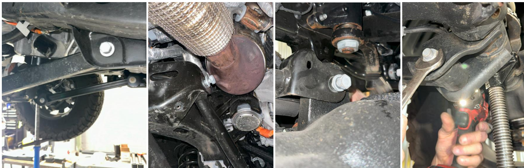
Figure 8: Lower/upper frame-side control arm bolts, and lower/upper axle-side control arm bolts
