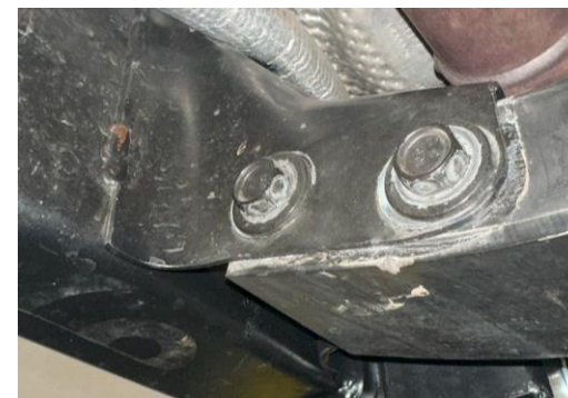
Figure 3: Cross-member bolts flipped around
