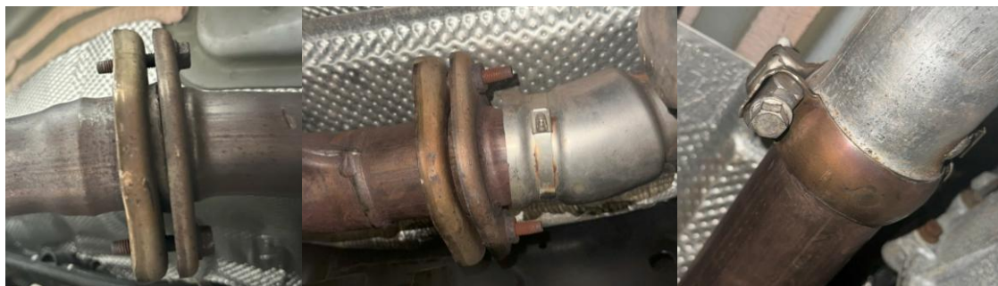
Figure 11: Exhaust section flanges and clamps
